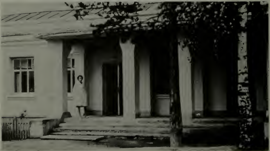
Administration Building, Mental Hospital #14 at Ramenskoy Village.
